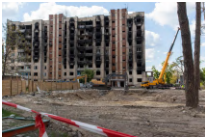
Fire Incident Inspection
